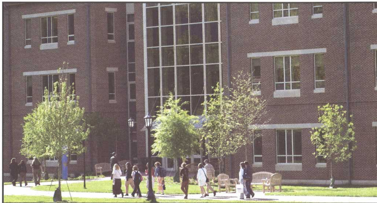
The Science Center overlooks the sunny South Quad, a new open space on campus flanked by Alston Campus Center, McCain Library and Campbell Hall. The quad is located on the site of the old field hockey field.
