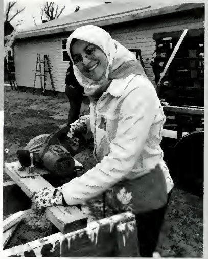
Workin' Hard: Kaleh Karim saws a board that will be used to build the house.
