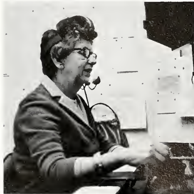
m. whitley, switchboard
