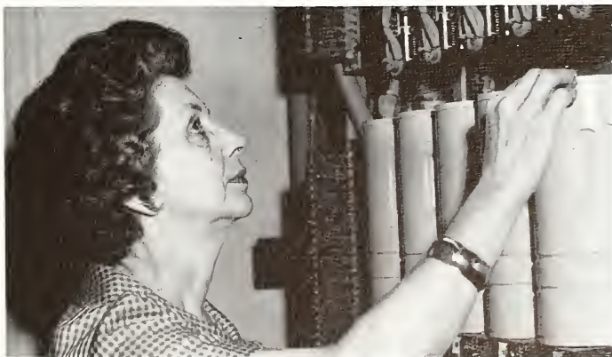
Mary Whitley inspects the many wires of the switchboard.
