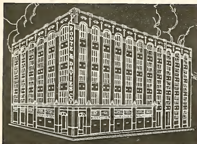
Offices and Store
