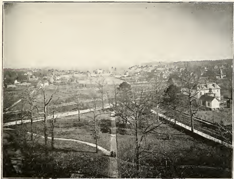
VIEW OF DECATUR LOOKING NORTH FROM THE TOWER
