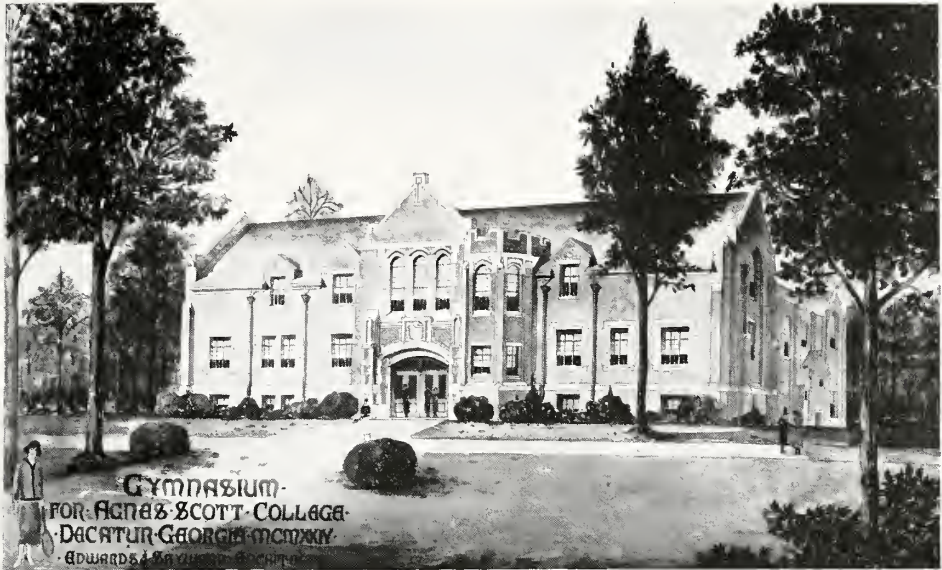
NEW GYMNASIUM-AUDITORIUM—FRONT VIEW.
