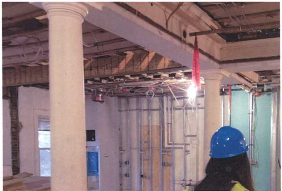
Rebekah Waltz unfurnished during construction. Photo courtesy of Karina Leung '18.
