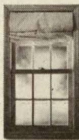
If all gas-heated homes were properly weather stripped we'd save enough natural gas to heat 4 million homes.
