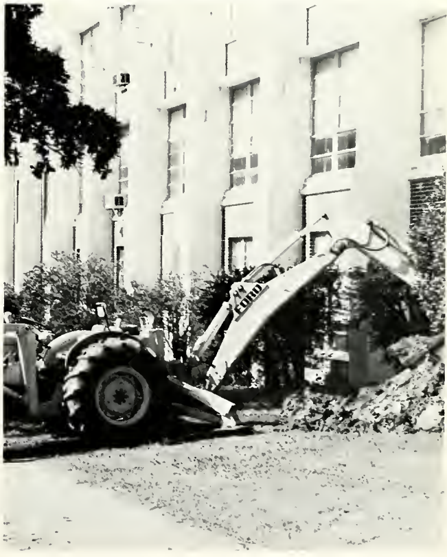
Repairs are made to broken underground pipes.
