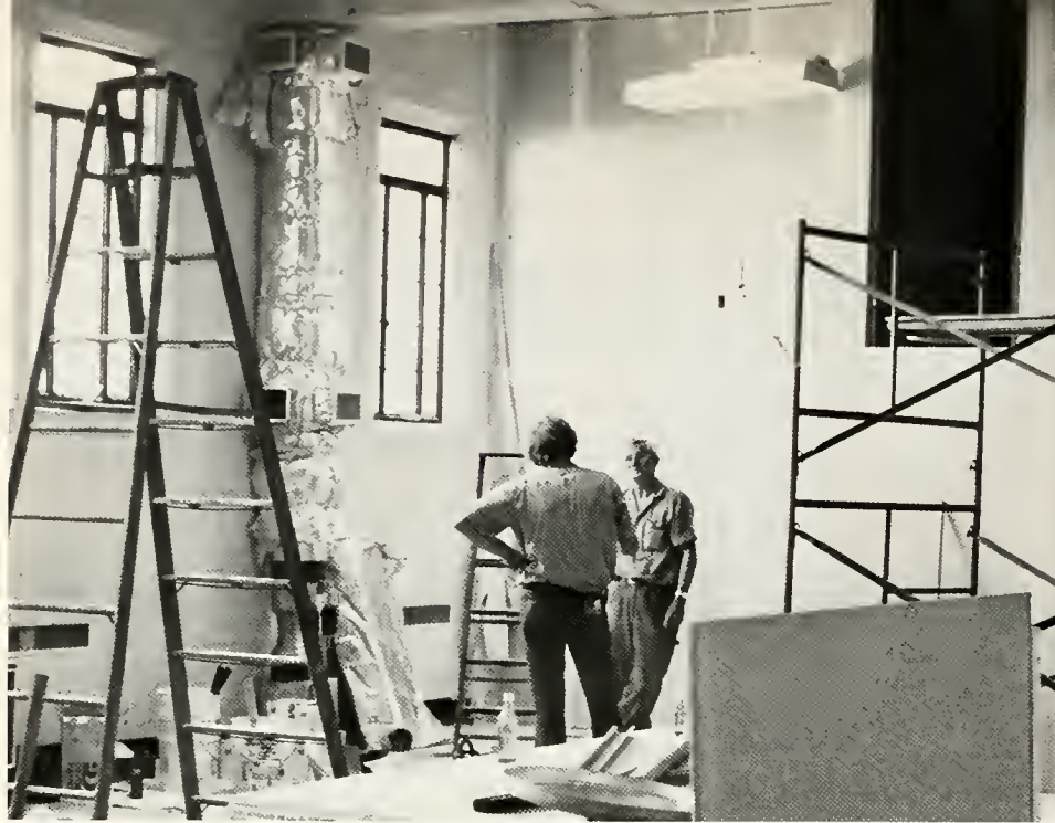
Workmen prepare to convert a high-ceilinged basement room in the Library into rooms on two different floors.
