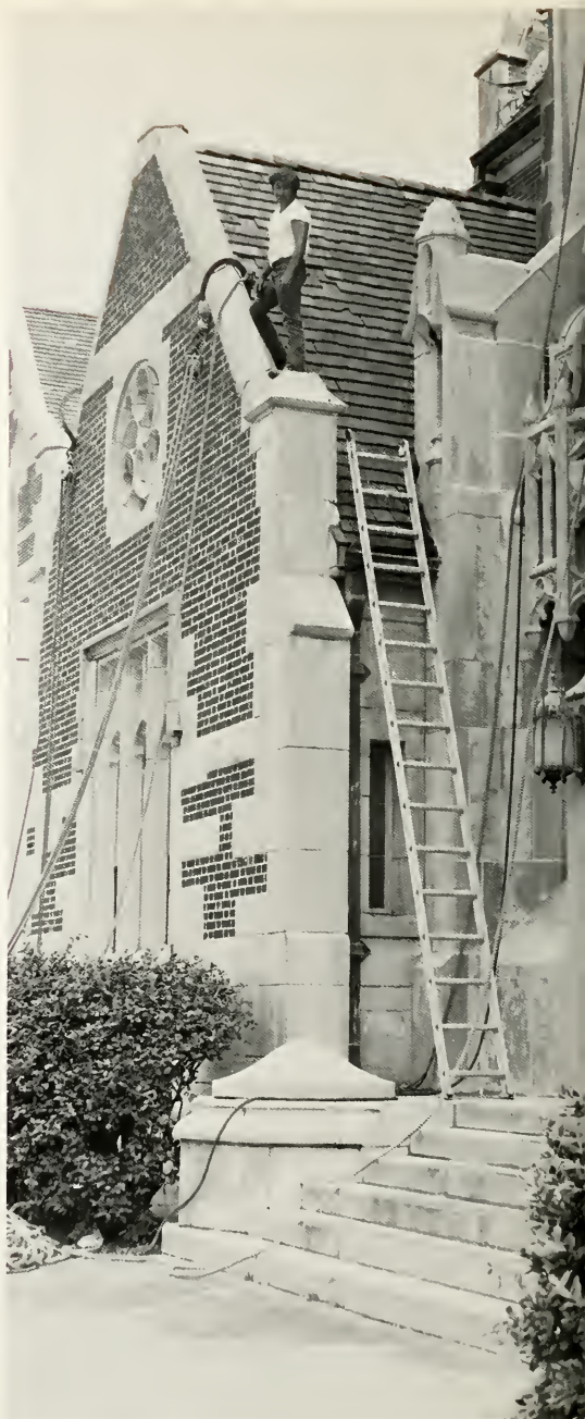
Buttrick receives weatherproofing and roof repairs.
