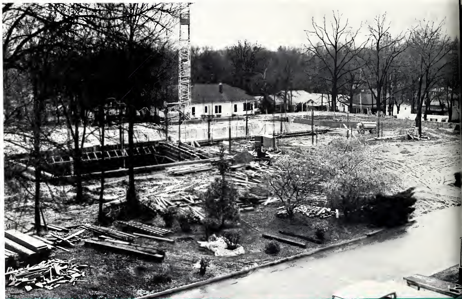
Early spring rains have made Georgia red clay mud at the site of the Dana Fine Arts Building.
